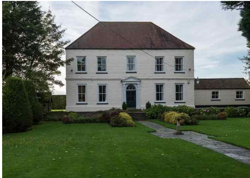
Manor House Farmhouse, Strensall
