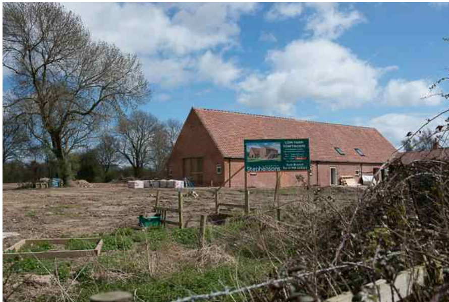
Towthorpe - The conversion of agricultural buildings
