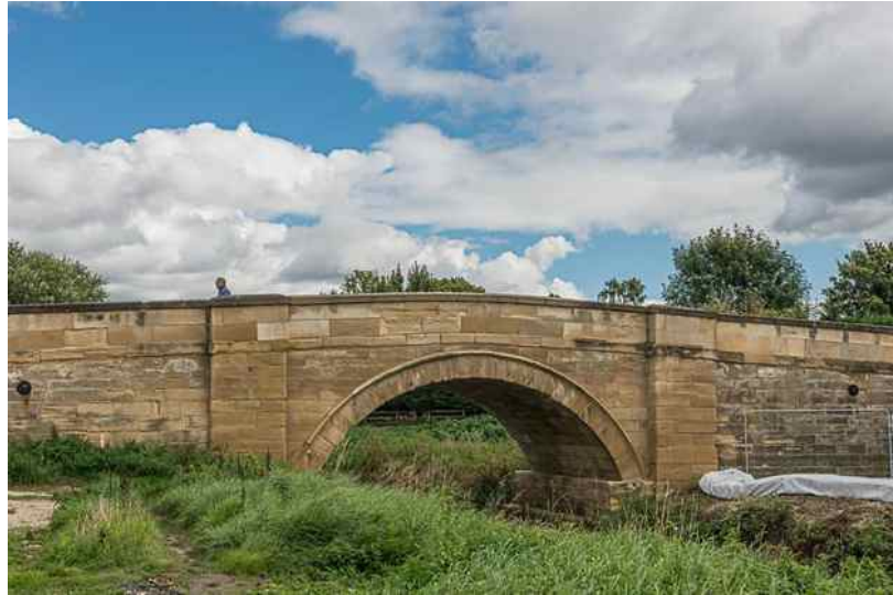
Strensall Bridge - John Carr's Bridge
