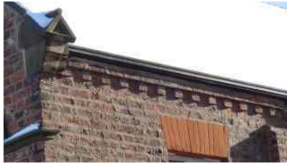
Decorative Banding and Brick Cambered Lintel
